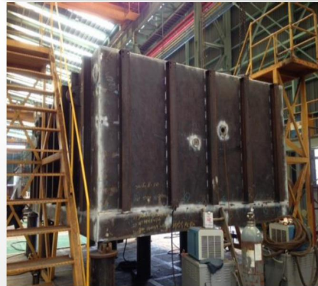
LUBE OIL SYSTEM
